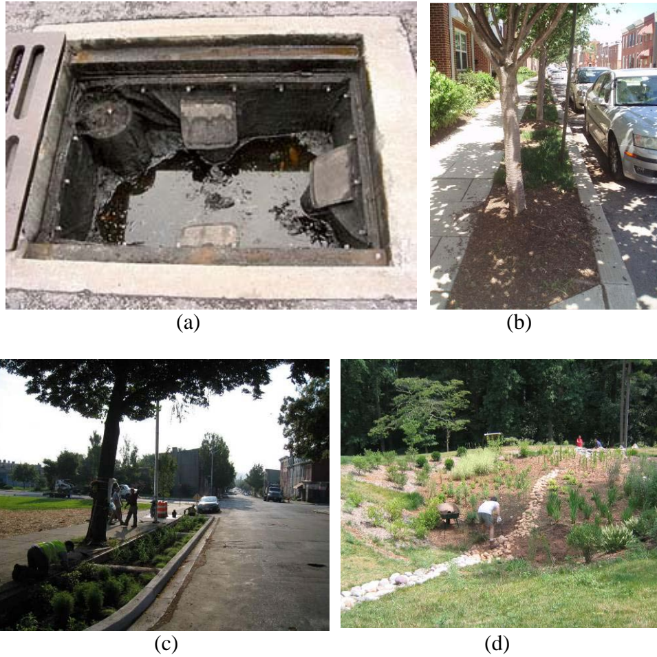
Figure 4.8. Street retrofit designs. (a) Proprietary catch basin insert installed at the Naval Station in Mayport, FL. (b) Recommended tree planting design in Canton, Baltimore. (c) Example of a street stormwater “bump-out” in Watershed 263, Baltimore. (d) A bioretention practice in a city park in Charlottesville, VA.
